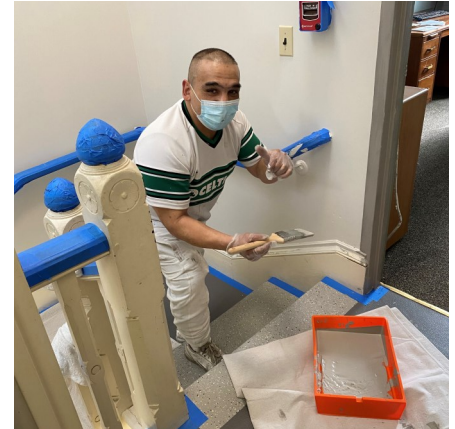
Elias Perez doing a masterful painting job.
