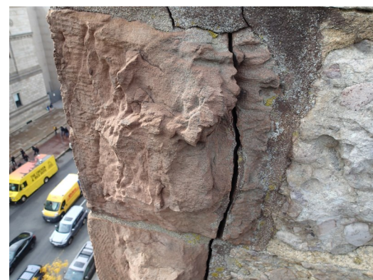
A crack at the one of the corners that needs to be rebuilt
